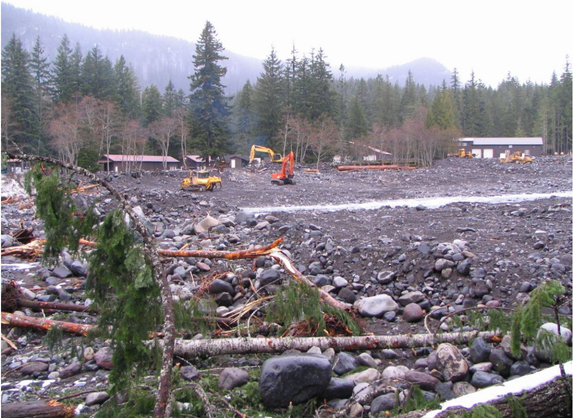
▲ FIGURE 6.9 Bulldozers and heavy equipment channelizing and altering the natural active channel of the Nisqually River at Longmire following November 2006 flooding. (Photo: Scott Beason, 11/21/2006)
