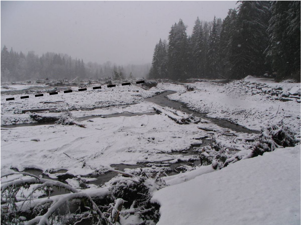
▲ FIGURE 5.11 Damage to Sunshine Point Campground. Dashed line approximates former river/campground boundary. Longmire-Nisqually Road curves on the left (Photo: Scott Beason, 11/23/2006).
