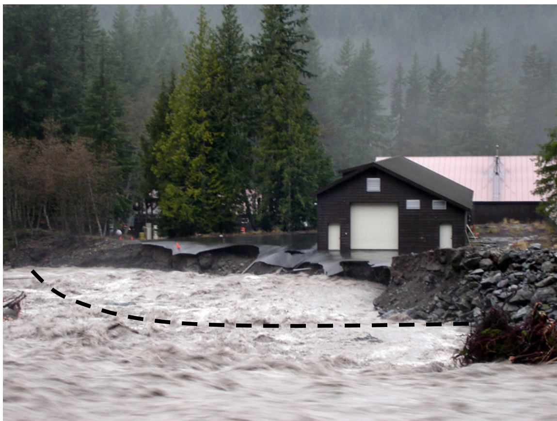
▲ FIGURE 5.1 Damage to Emergency Operations Center, levee and parking lot from flooding in November 2006. Dashed line shows approximate former levee boundary. (Photo: National Park Service, 11/17/2006).
