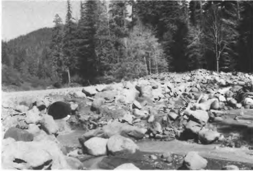
Figure 12.--Debris-flow deposits of September 8, 1992 on Westside Road, near confluence of Fish Creek with Tahoma Creek (river km 5.0). The culvert diameter is about 1.5 meters.
