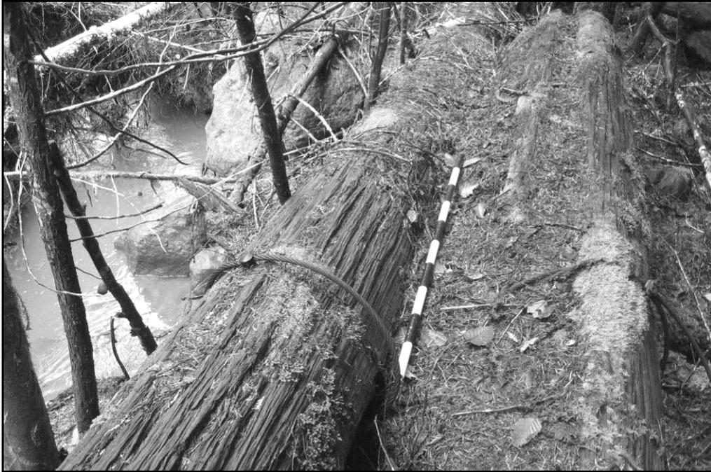
**Figure 28. Close up of logs with cables anchored with railroad spikes.** Boulders that would have formed the creekside portion of the levee have been displaced by 2006 floods.
