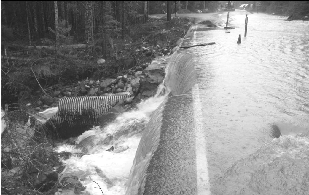
**Figure 22. Small Culvert Extends from the center of a Ten-foot Diameter Culvert Built in the Mid-1950s.** Photo of receding flood water taken in November 2006.
