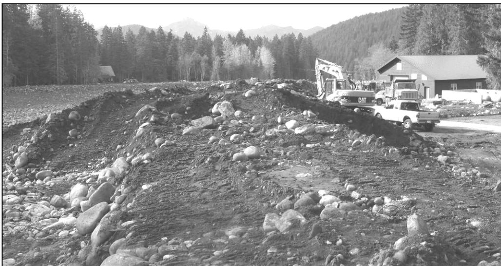
**Figure 33. Buried Concrete Floodwall and Levee Under Construction in 2007. EOC on the right. Community building and realigned river bank across the Nisqually in the background.**
