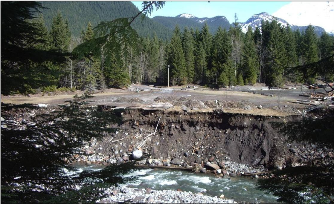
**Figure 17. Eroded Nisqually North Bank at Kautz Service Area.** Helipad near photo center. Wood storage area at photo right. Circa one meter artificial fill at the surface, with eroding metal, wood, and other buried debris scattered on the exposed cut-face.
