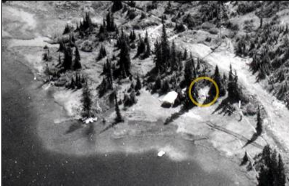
Figure 17. Close-up of Figure 9 showing log stockpile (circled in yellow) from FS2005-23
