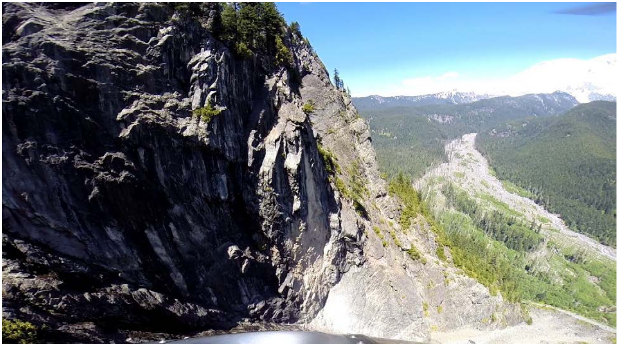
Figure 4: Go-Pro screen grab of helicopter view of source area (center of photo) and downslope debris fan (lower right) (NPS/Scott Beason).
