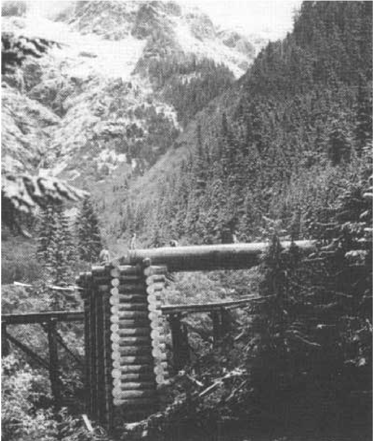
Figure 2.8. Bridge over the North Puyallup River under construction in 1934; a representation of the time and place where local wilderness values abruptly changed. Source: National Park Service, http://www.nps.gov/history .
