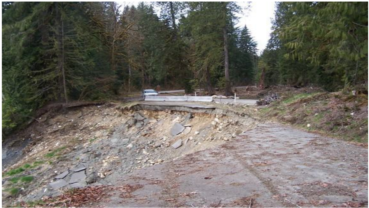
Figure 3.5. Washout at milepost 12.6, Suiattle River Road. Scheduled for repair beginning in 2013. Source: US Forest Service EIS.
