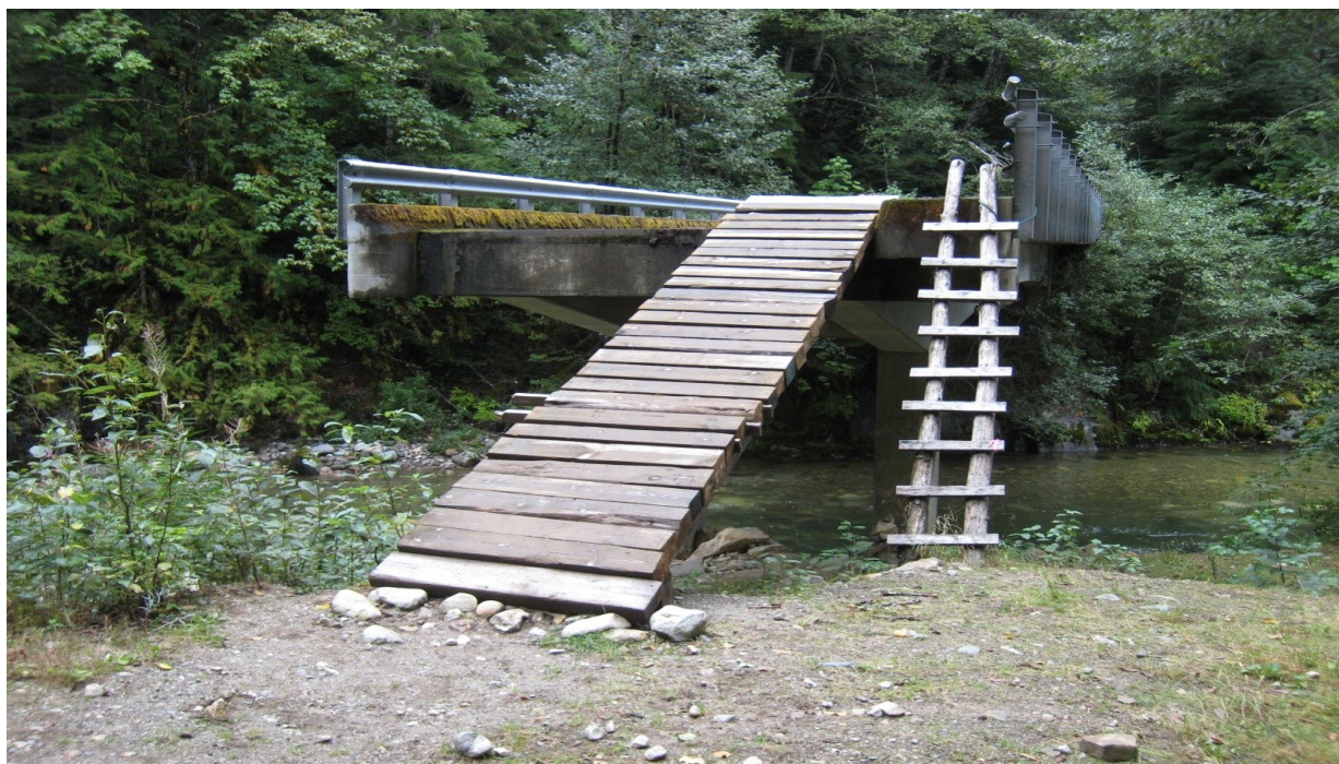
Figure 3.9. Former automobile bridge on Suiattle River Road near Downey Creek, milepost 22.8—a ten mile walk from the car. Photo by author.
