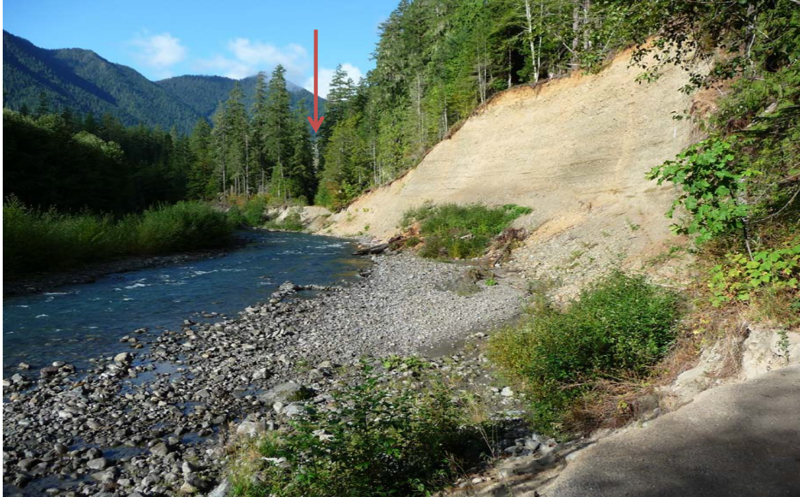
Figure 3.1. The washed out section of the Dosewallips River Road in 2010. Note the road-break on bottom right and its continuation far beyond. Source: Olympic National Forest Dosewallips EIS.
