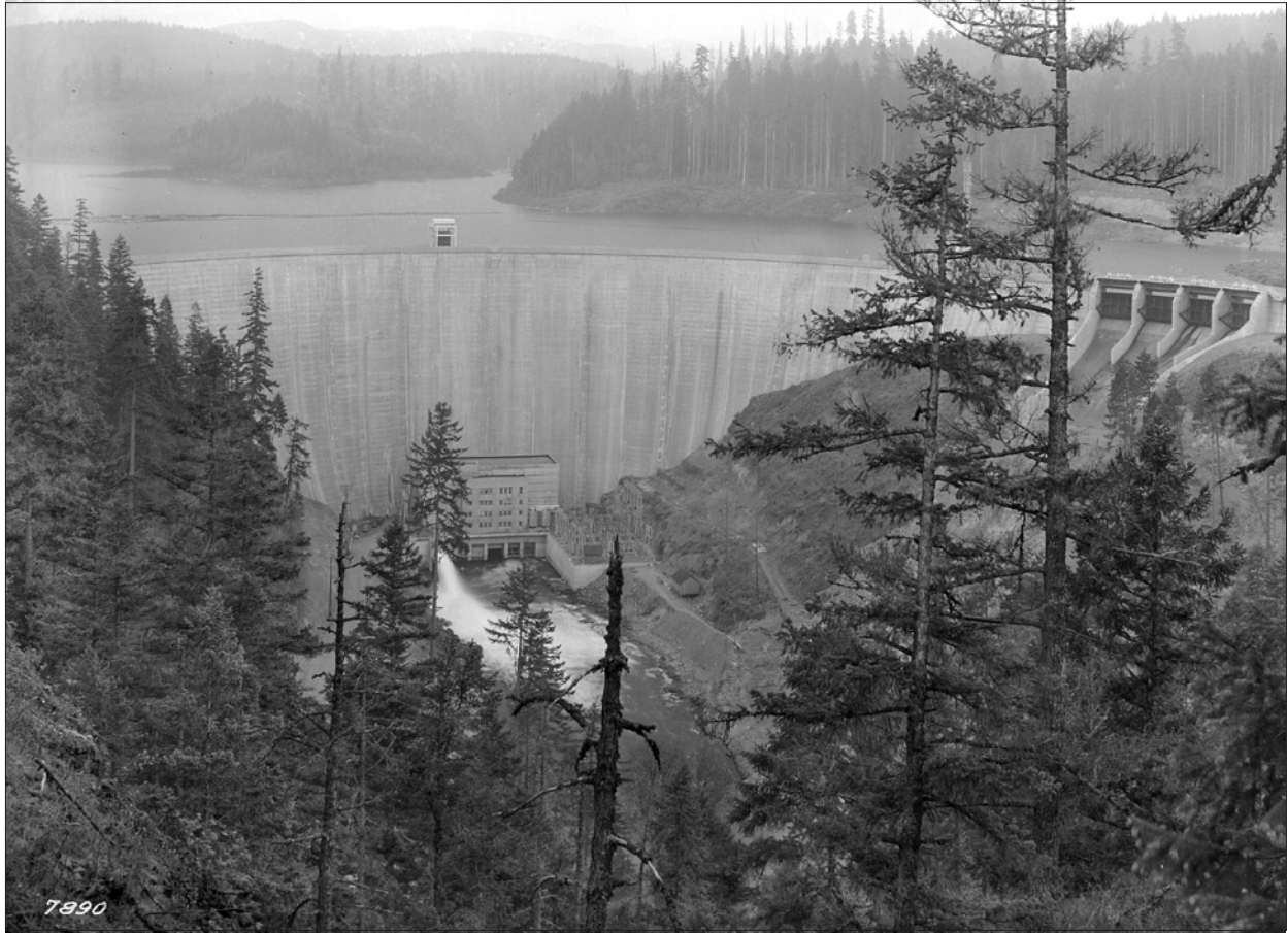
Figure 3. Alder Dam on the Nisqually River, Washington. (Courtesy of Tacoma Public Utilities, Tacoma Power, date unknown.)
