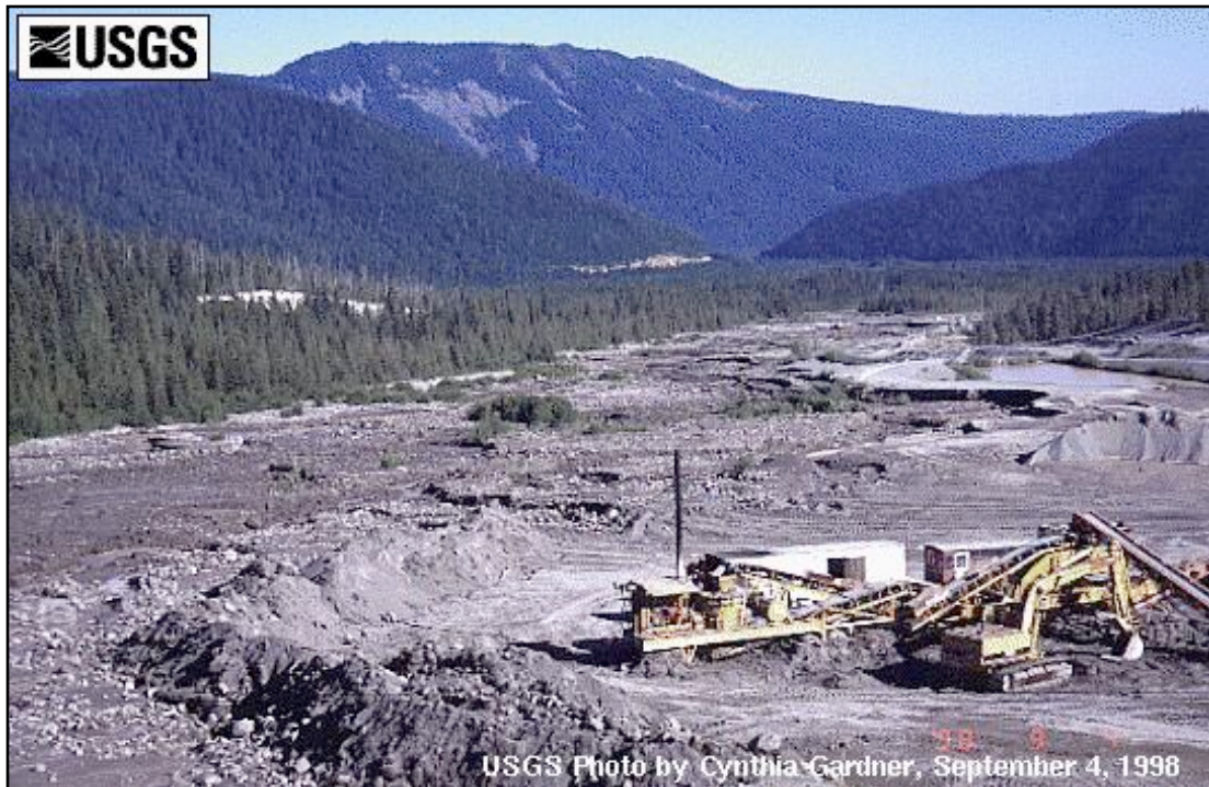
Figure 1.15. The Oregon Highway Department repairing the White River Bridge after a debris flow in 1998 tore it out.
