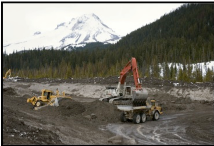
Figure 1.6. Highway 35 repair after a debris flow washed out the bridge over the White River.
