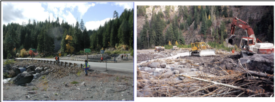
Figure 1.12. Polallie Creek on Mt. Hood before and after a debris flow. Courtesy Amit Armstrong.
