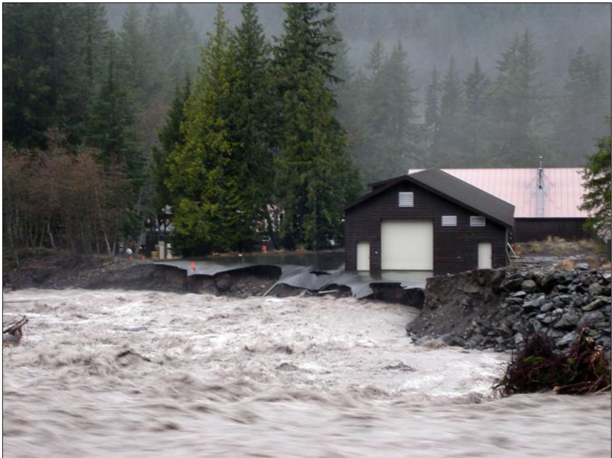
Figure 9: Bank erosion and damage to park infrastructure during the November 2006 flood at Mount Rainier. Photo taken at 9:39 AM on November 7, 2006, after the peak of the flood. Photo: National Park Service.
