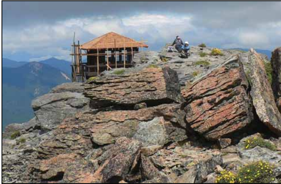
Mount Fremont and Gobbler’s Knob Fire Lookouts now have roofs and interior restoration will continue into 2008.
