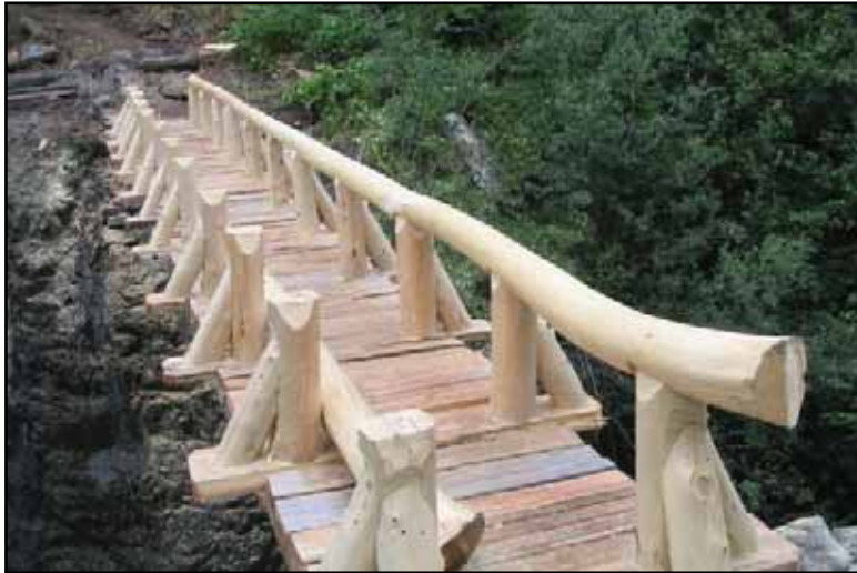
With the help of volunteers and park crews, six backcountry bridges, have been replaced, such as this one over the North Puyallup River.
