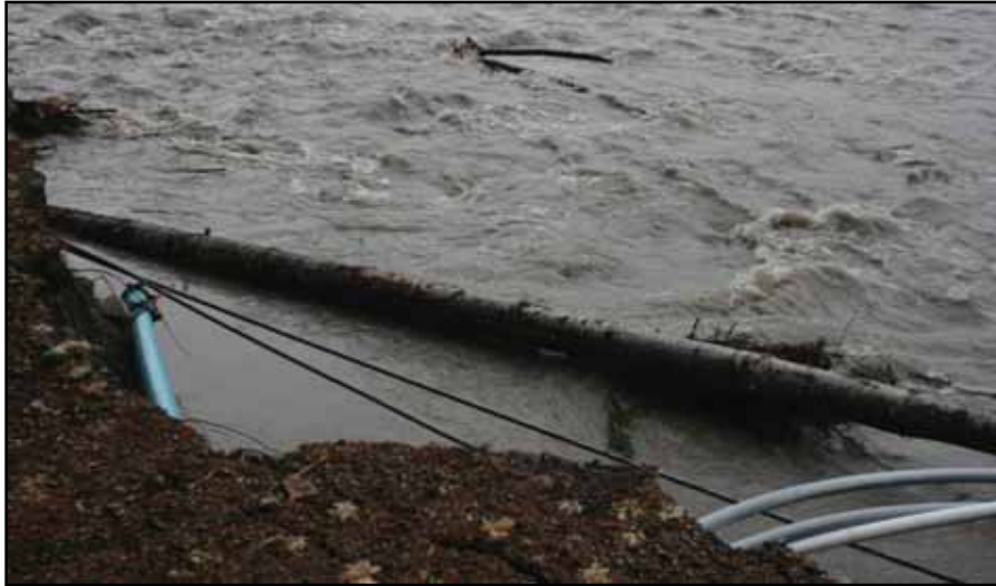
The park's buried power line was destroyed for a length of 1200 feet at Sunshine Point, shorted out at Kautz Creek and exposed by erosion in two other places. The overhead line to the water treatment plant at Longmire was also broken.
