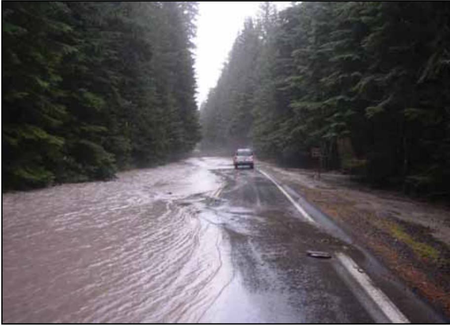
The White River now runs 12 feet above the elevation of Highway 410 for three miles.
