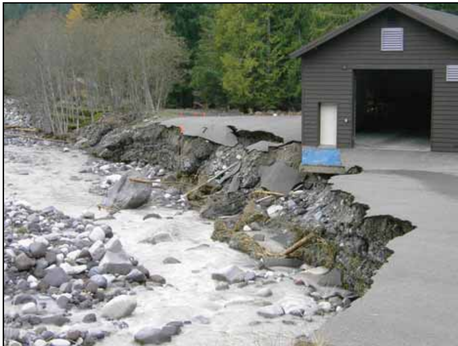
The Emergency Operations Center at Longmire was especially vulnerable. Sixty feet of levee and river bank eroded away during the storm, leaving one corner of the building hanging over empty space.
