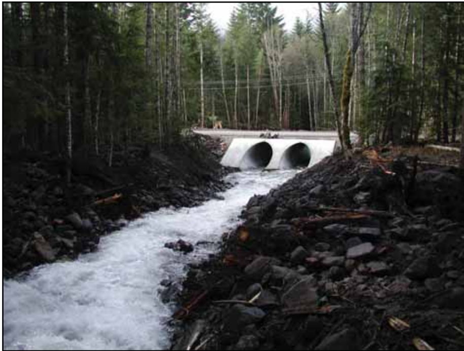
Two 12- foot culverts accommodate the new Kautz Creek channel at Nisqually Road.
