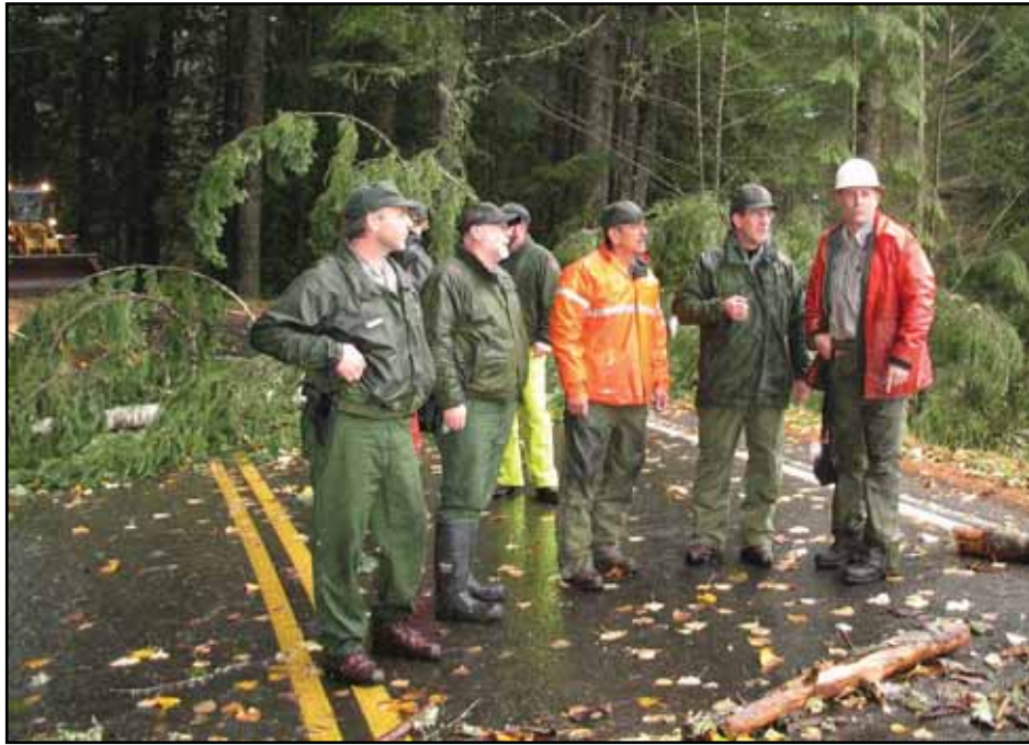
On Nov. 7, 2006, park staff began evaluating the damage and initiating repairs.
