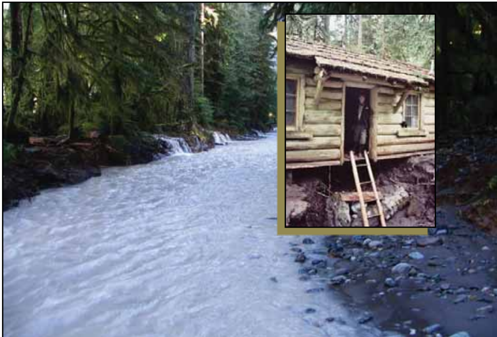
More than two miles of road were destroyed along the Carbon River. Ipsut Creek cut a deep channel directly beneath the historic Ipsut Creek Patrol Cabin.
