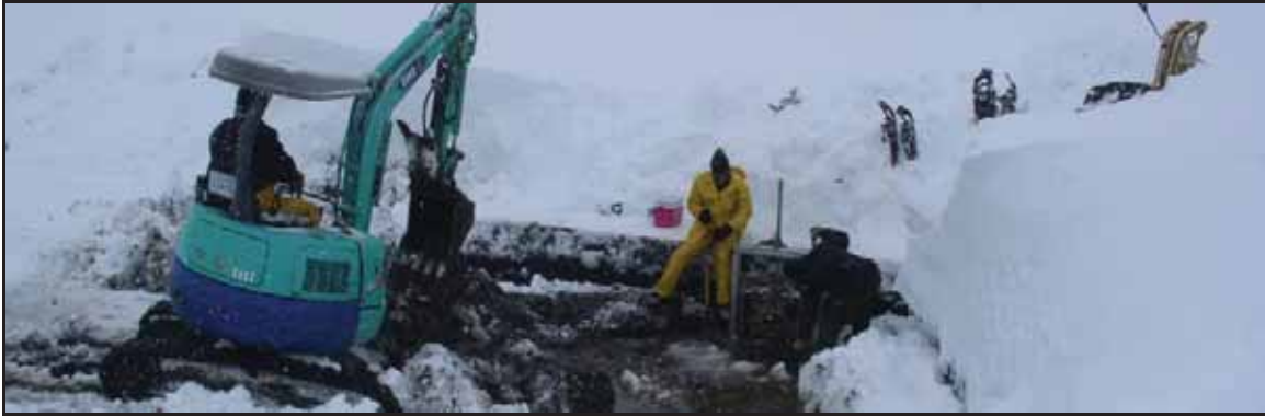
Power, sewer and water utilities were restored, despite 10 feet of snow on the ground at Paradise.
