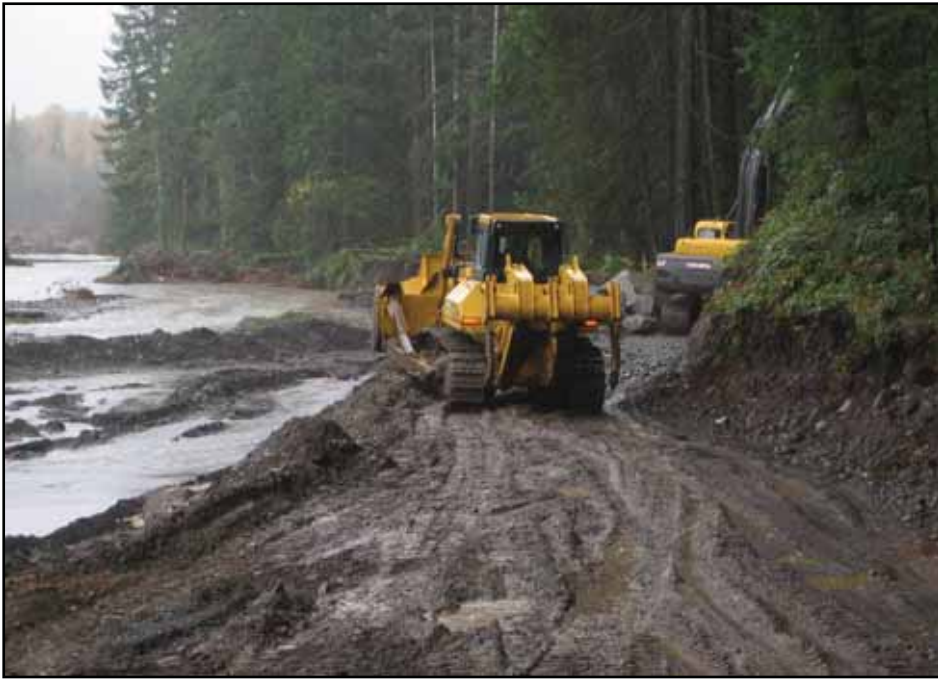
At Sunshine Point, construction began on a replacement road on November 8, 2006.
