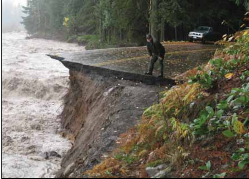
Sunshine Point Campground was gone, along with 200 yards of road.
