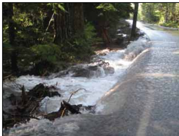
Kautz Creek left its channel more than a mile upstream from the park road. It flowed through the forest and then over and under the park road 200 yards east of the bridge.
