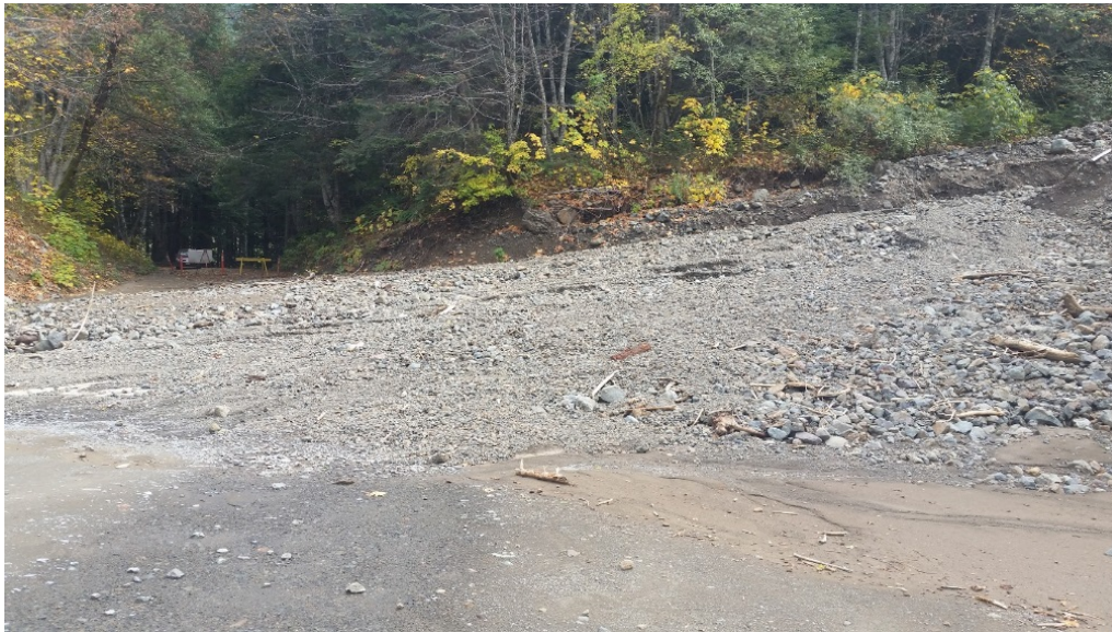
Figure 8. October 10th Dry creek debris flow covering the Westside Road (photo NPS).
