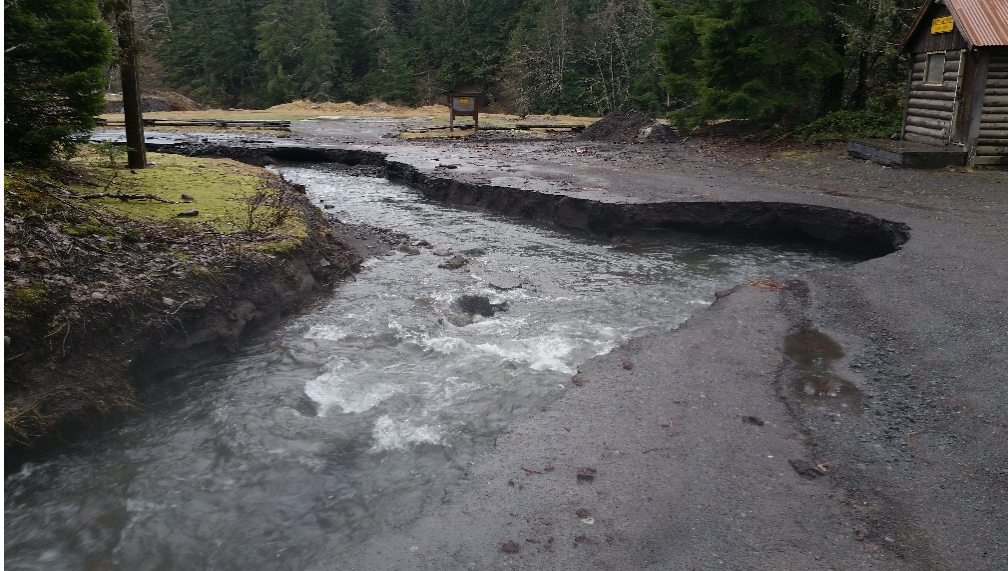
Figure 9. February 14th Kautz creek avulsion damaging the maintenance area (photo NPS).
