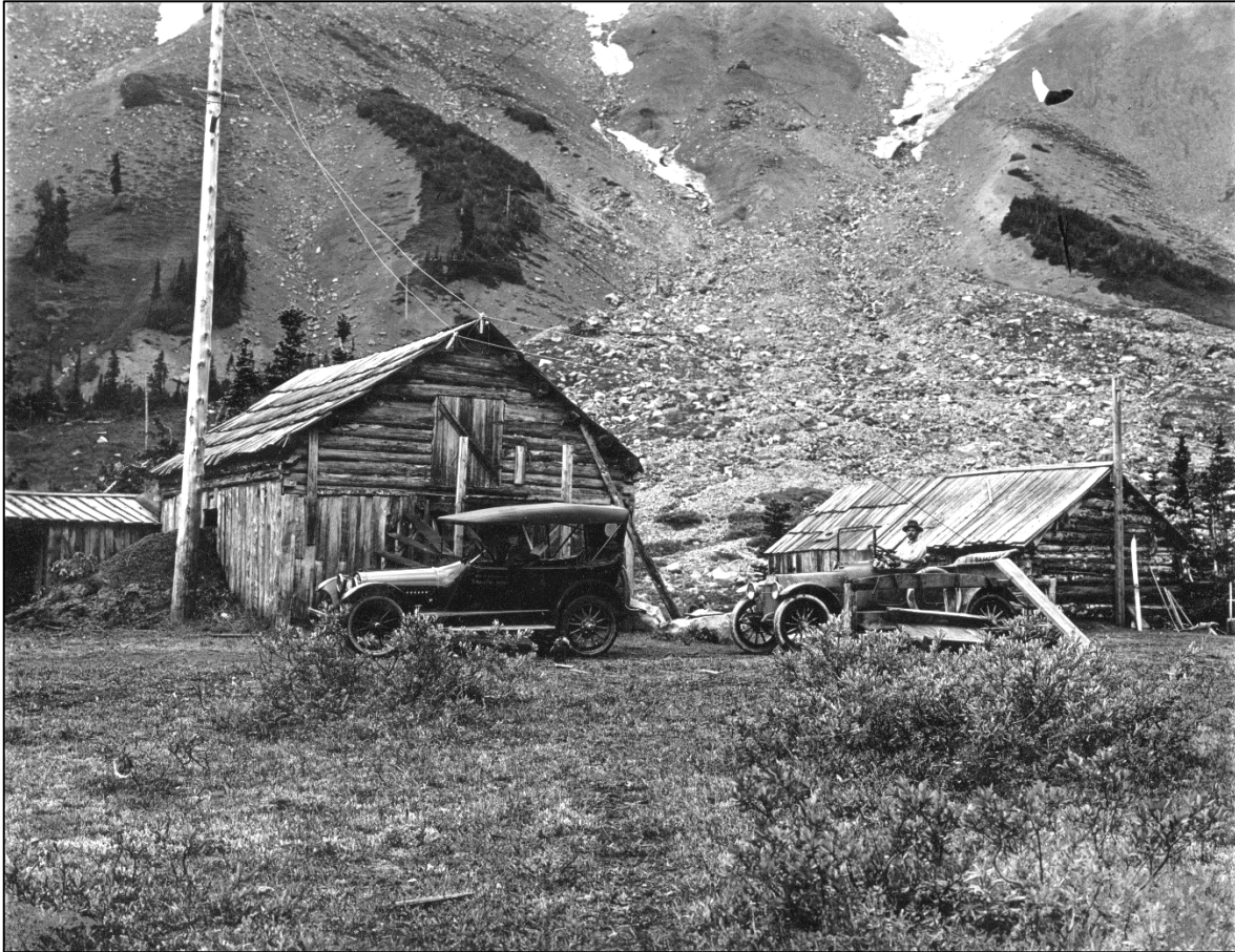
Figure 3.23. 1918 Photograph of Lower Camp's Barn ( left ) and Cabin ( right ). Barn with rear addition on the left with mound of manure and/or coal slag at side opening. Across the Inter Fork, the aerial ore tram is visible extending diagonally upslope behind the barn to Snowflake Lode. (MORA Archives)
