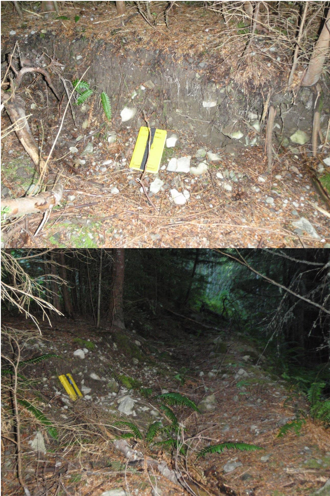
Appendix Figure 8: Deep-Seated Hazard Example. Upper photo shows an example of vertical offset above a bench within the hazard zone. Lower photo is a view of the same location looking W. These are just one example of benching and cracking that occur across this 280 meter zone of trail.
