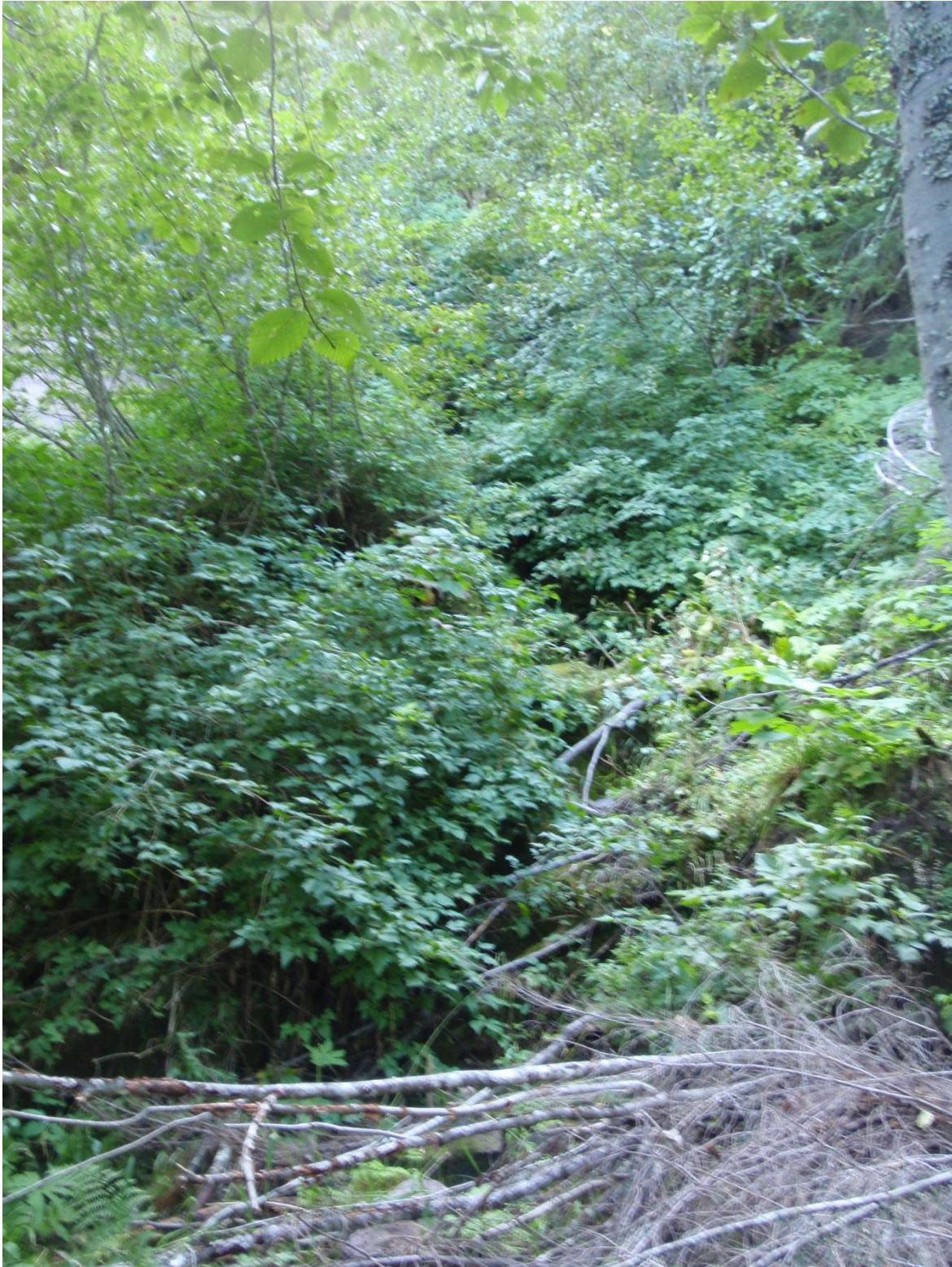
Appendix Figure 3: Point 10 Channel. Photo detailing the smaller clogged channel contacting the trail from upslope at point 10. This channel is constricted at its base and produces some ponding near the trail.
