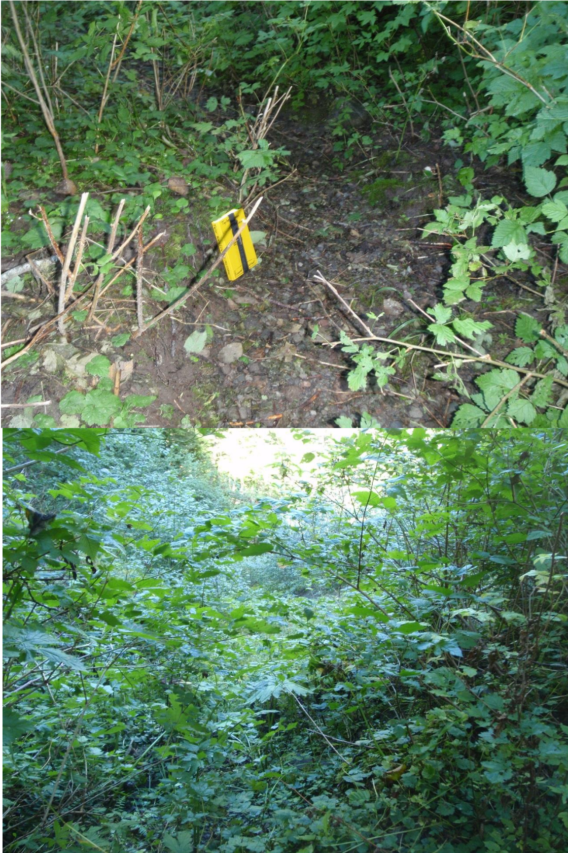
Appendix Figure 6: Point 21 Conditions. Upper photo shows the surface scouring that exists near the point 21 colluvial hollow headwall. Lower photo shows the condition of the interior of the hollow. The scour in the upper photo does not lead into the hollow.
