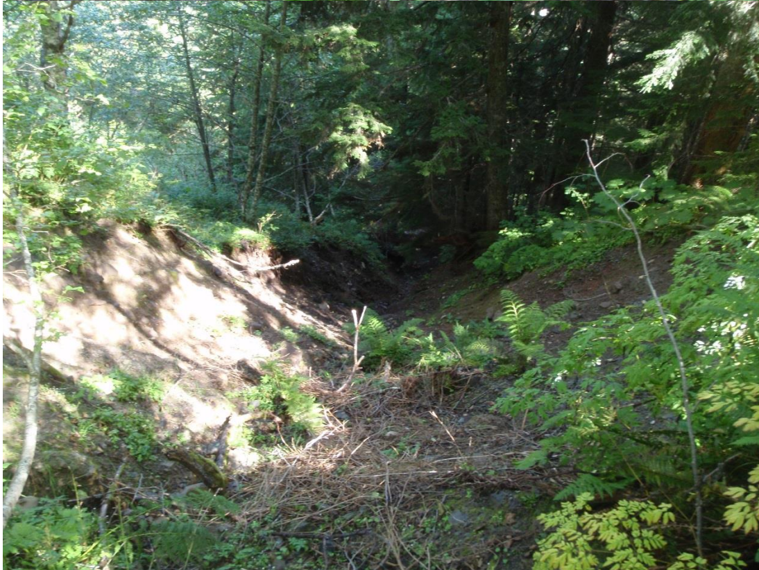
Appendix Figure 2: Photos of Point 9 Concerns. Upper photo shows the entrance to the point 9 culvert that has no exit. Lower shows the point 9 colluvial hollow emanating from the fill slope.
