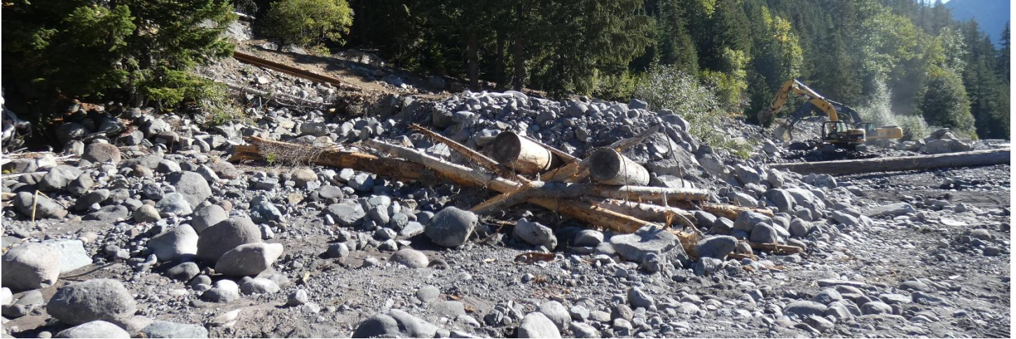
Figure 4: Photo showing the fully constructed condition of barb 4. The two chainsaw cut logs are installed with the barb as ballast, while all other wood was taken from the floodplain and strategically placed along the barb face to slow high flows (Photo: NPS/Taylor Kenyon).
