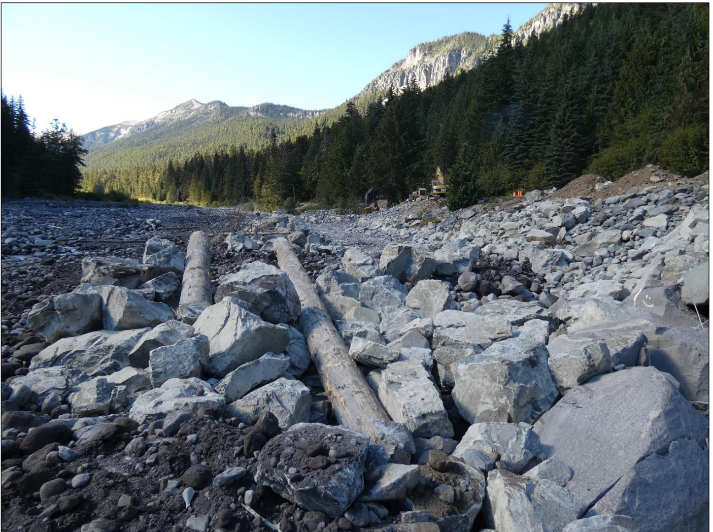
A partially constructed barb 6 at the end of a work day. View looking upstream in the White River watershed (Photo: NPS/Taylor Kenyon).
