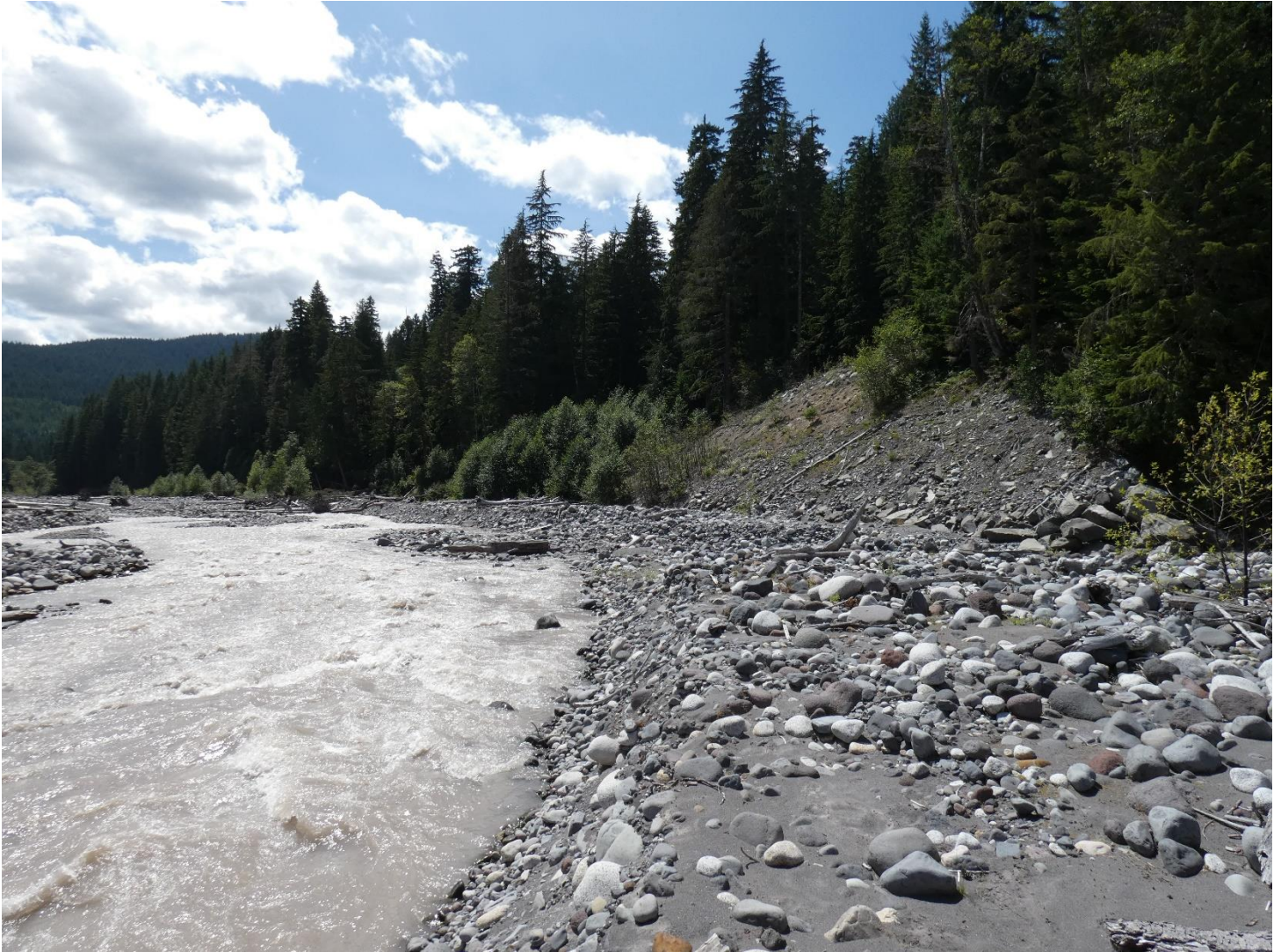
Figure 5: Milepost 5.3: Anthropogenic riprap on the right and the road is right on top of it as the tree line. (Photo: NPS/Jessica Bersson)
