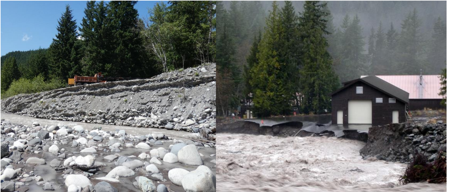
Figure 7: Left: Longmire levee June 2019 river right eroding away with equipment parked on top (Photo: NPS/ Shelby Cutter). Right: 2006 flood event at Longmire Emergency Operations Building (Photo: NPS).
