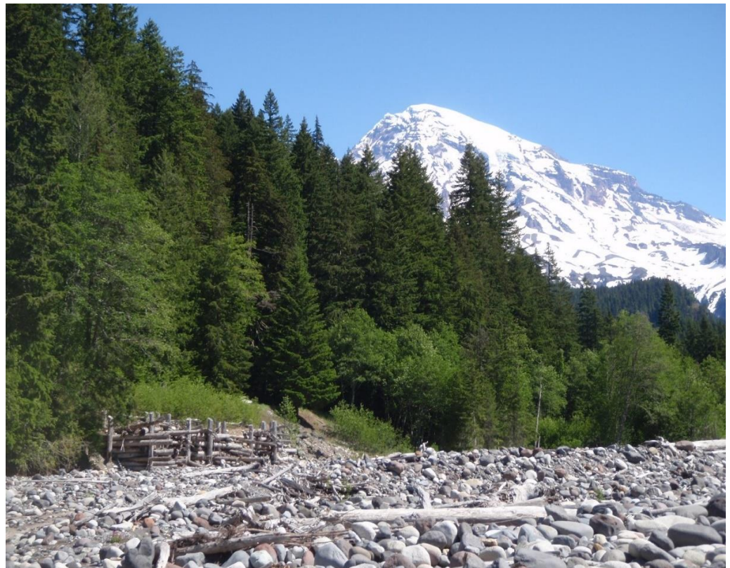
Figure 6: Milepost 6.0: Looking upstream at the engineered logjam (ELJ) placed in 2010. The road is directly above the ELJ. (Photo: NPS/Shelby Cutter)
