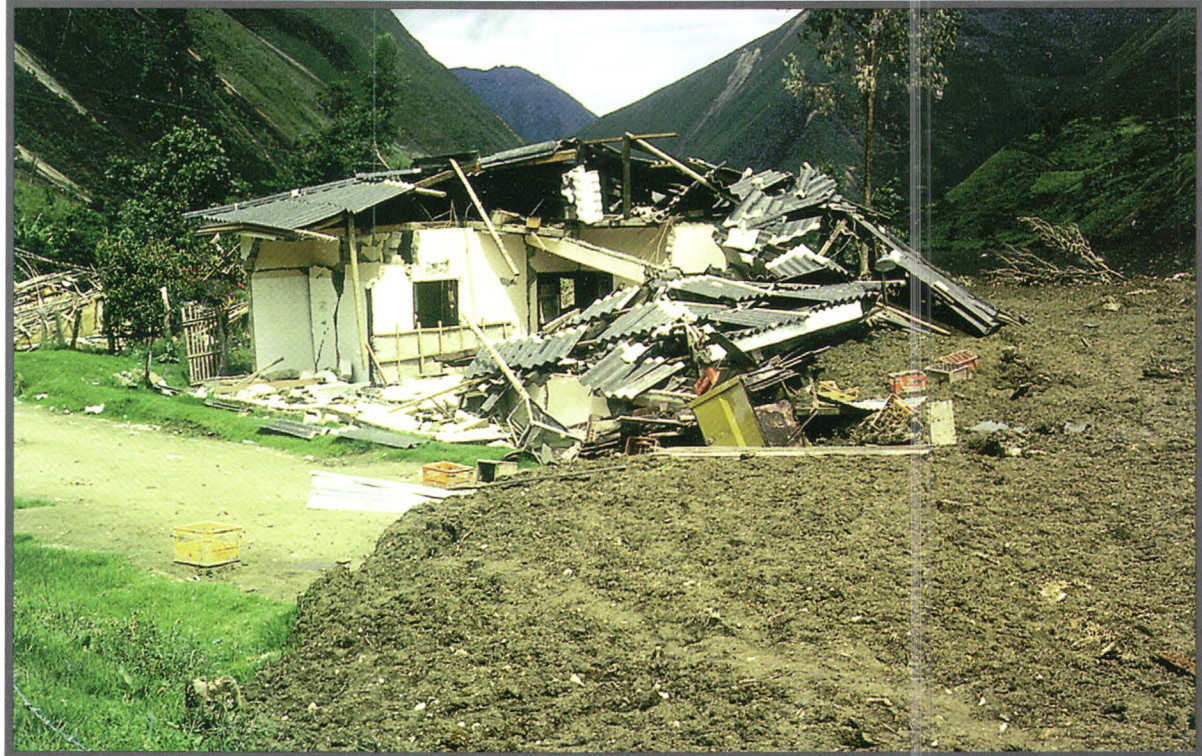
Figure 7. Margin of “la avalancha” looking downstream where it inundated the only remaining street. Deposit thickness is 1.2 m. Location shown by right pointer in figure 5.
