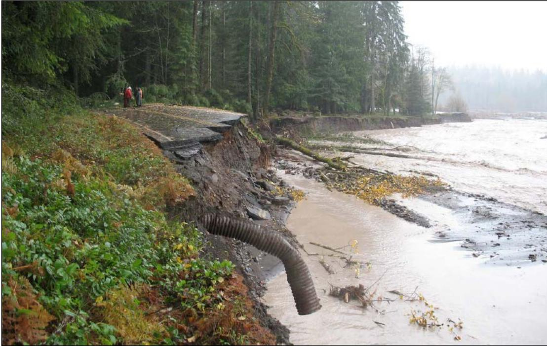
**Figure 14.** The Nisqually Road and the site of the former Sunshine Point Campground, which was destroyed by the 2006 flood (NPS photo).
