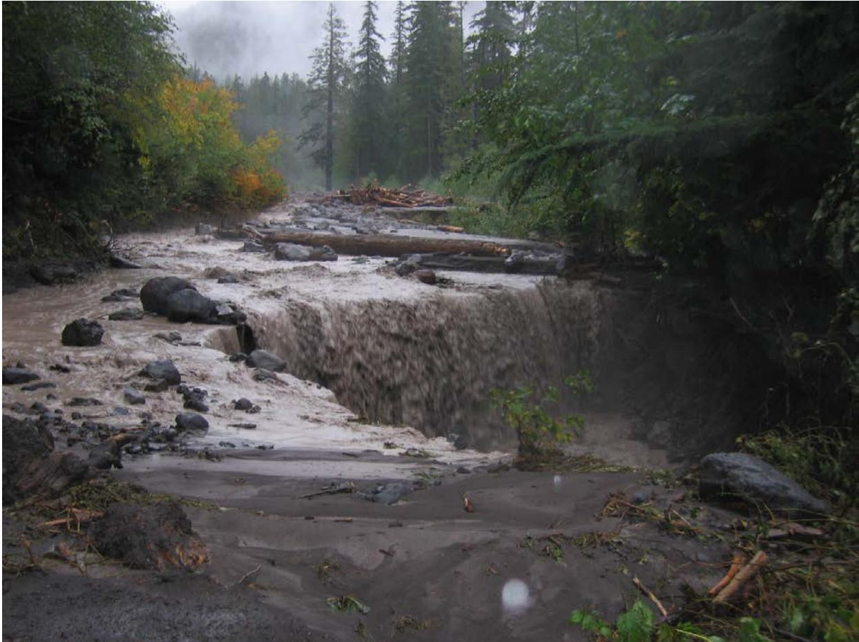
**Photo 3:** Damage to the West Side Road during the September 29, 2005 flood at Mount Rainier (NPS Photo).
