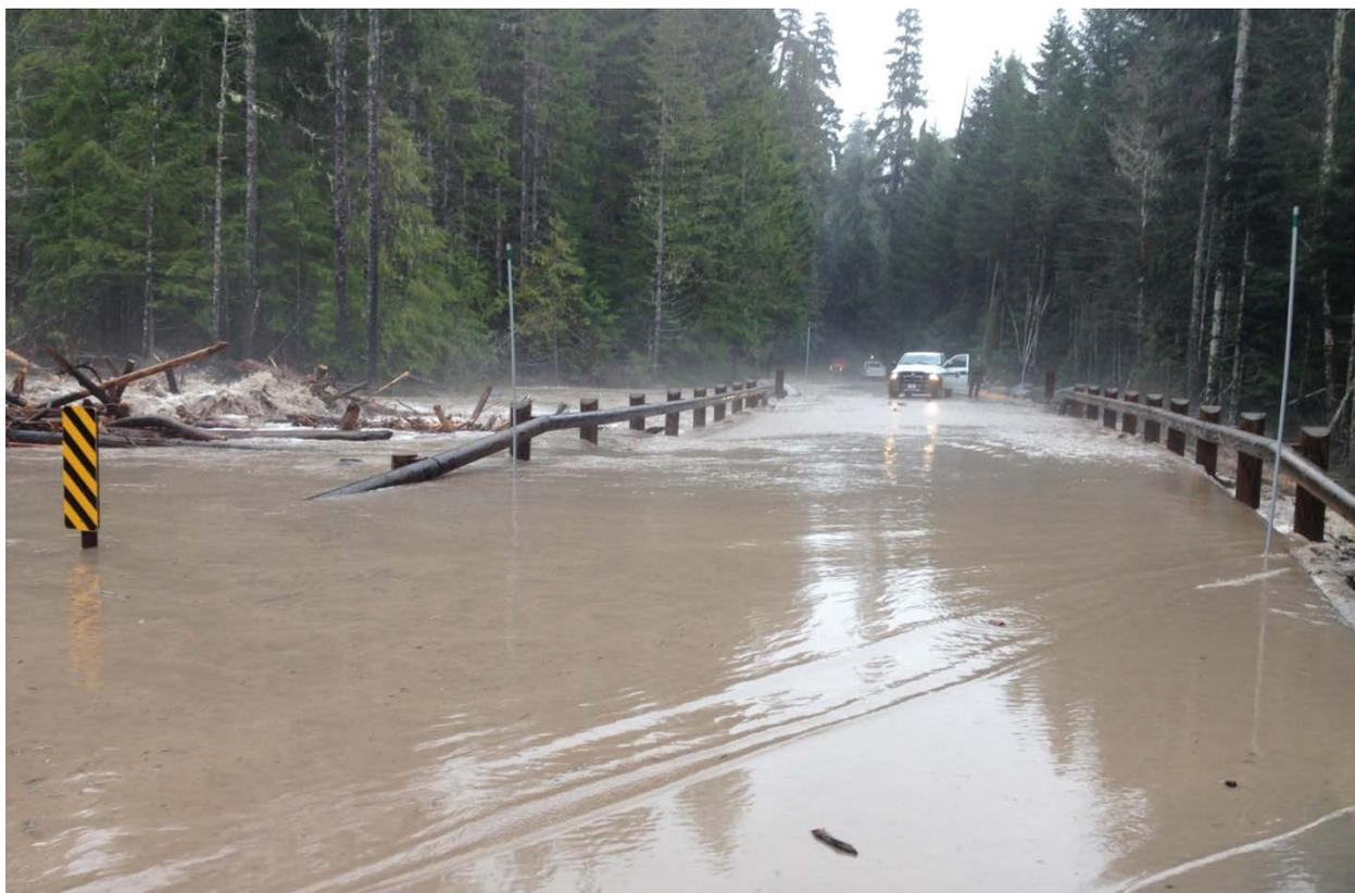
**Figure 20:** Floodwaters overtopping the Kautz Creek culverts (NPS Photo).
