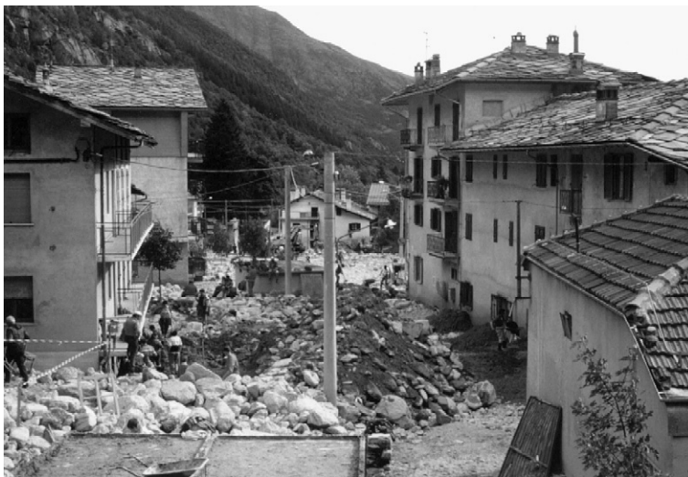
Fig. 9. Coarse debris accumulation in the village of Forno Alpi Graie, following the 24 September 1993 debris flow (site 1). The deposit was up to 4 m thick.
