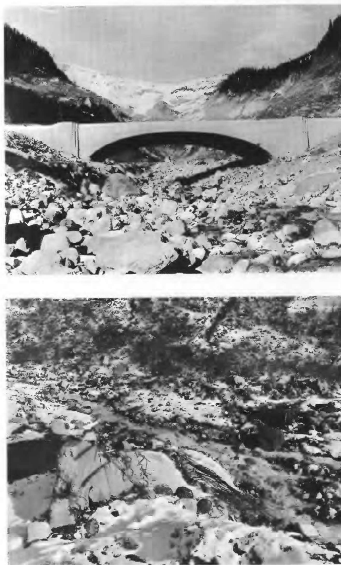
FIGURE 2.—Nisqually Glacier bridge before and after the flood of October 25, 1955. In the earlier view (above) the bridge is seen as it appeared soon after its construction in 1936. The terminus of Nisqually Glacier is visible in the background. After the 1955 flood all that remained of the bridge were the broken abutments and exposed reinforcing bars seen in the latter view (below). The large boulders on the far bank were left by the flood. Photographs by M. K. Potts, National Park Service.
