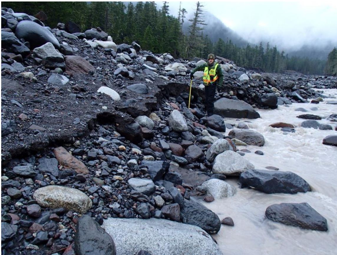
▲ Figure 2. Field evidence of high flow in the form of a trim line near Cougar Rock along the Nisqually River, upstream of Longmire. Similar trim lines were seen in the riverbed at Longmire and Lower Van Trump Hairpin. The flood did not originate in any tributaries of the Nisqually (Photo: Laura Walkup/NPS).
