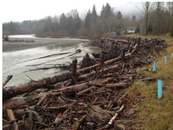
Fig. 6 ELJ installed as large wood revetment for bank protection along South Fork Nooksack River, Whatcom County, WA. Reference Module in Earth Systems and Environmental Sciences, (2018)
