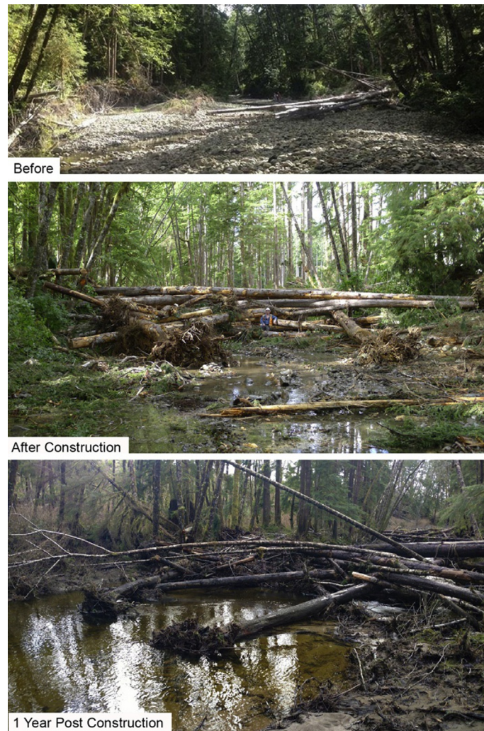
Fig. 19 Valley scale ELJ, pre-construction, post construction and 1 year afterwards. Hurst Creek, Jefferson County, WA.
