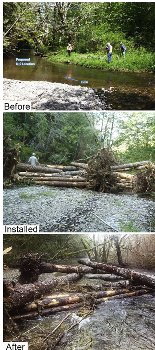
Fig. 14 Pre- and postproject conditions and 1-year post project conditions for ELJ retaining sediment in Big Beef Creek, Kitsap County, WA. View looking downstream.
