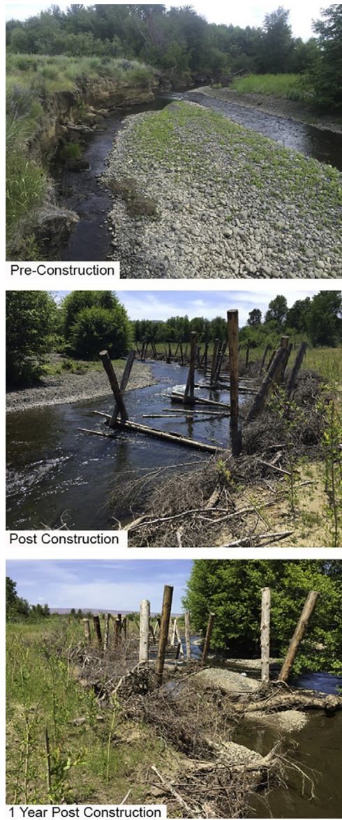
Fig. 8 ELJs installed in Toppenish Creek in 2016 to raise bed level, water levels and stabilize high banks lacking riparian trees. Yakima County, WA.
