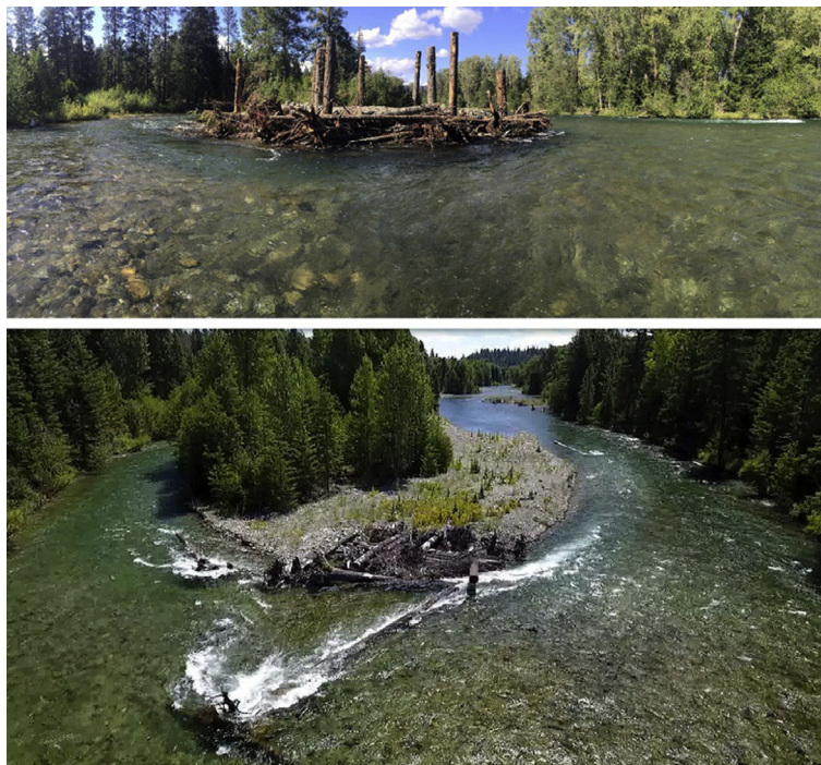
Fig. 17 Two examples of apex ELJs, Cle Elum River, Kittitas County, WA.
