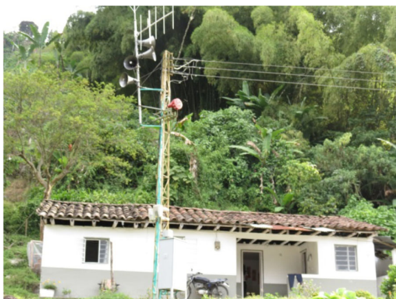
Fig. 7 In the upper center portion of the photo, a lahar siren system is visible mounted on a pole in the village of Viejo Rio Claro Chinchiná. Unlike in the US, local residents in Colombia have a personal role in lahar notification as they host and regularly test lahar siren devices installed beneath roof eaves and in public areas. USGS Photo by C. Driedger 2013
